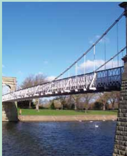
Civils Wilford Suspension Bridge
